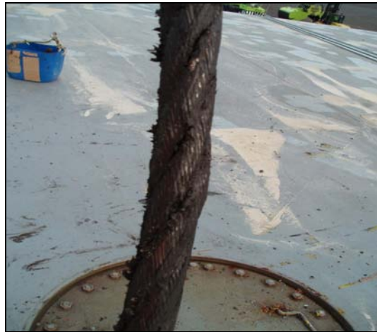
Photograph 6 – section of No. 4 hoisting wire
