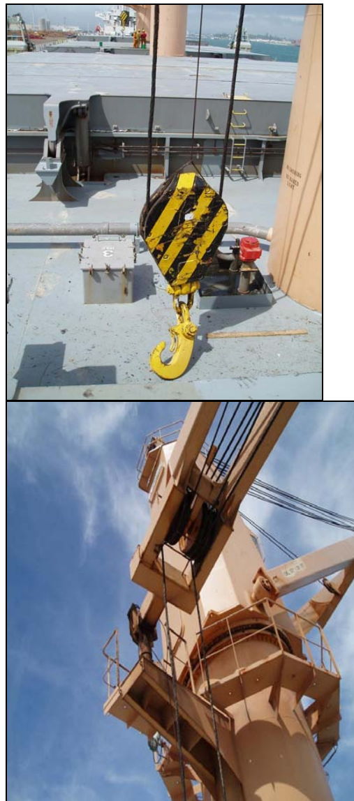
Photograph 5 – No. 4 jib and No. 3 crane pedestal
