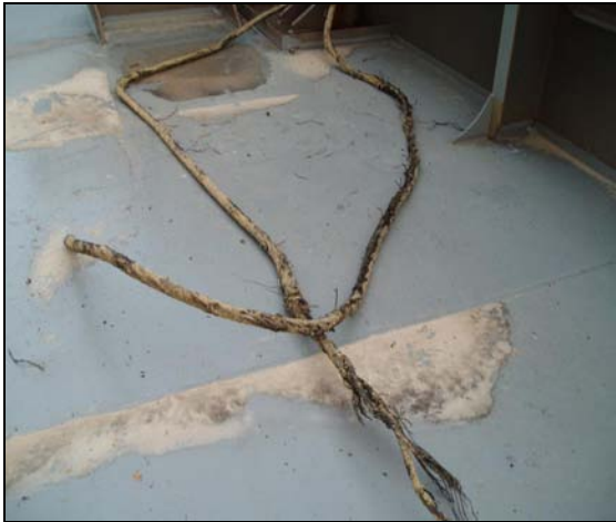
Photographs 5 - the broken hoisting wire rope
