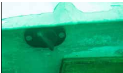
Photograph 15 The bungs were secure.
