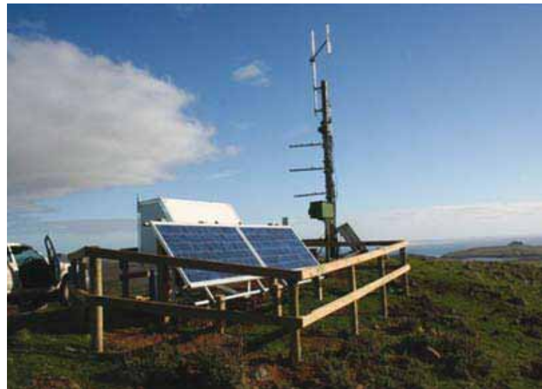
Construction work at the Rangitihia radio station.
