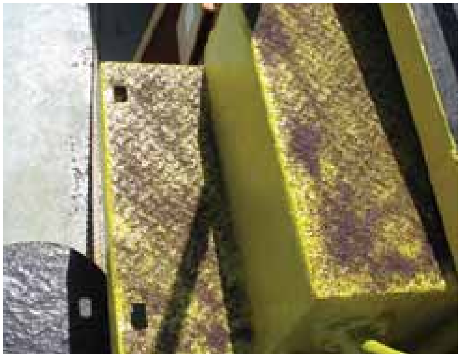
▲ DETAIL SHOWING NEW NON-SLIP SURFACE. ▲ REPAINTED STEPS AND NEW GANGWAY BRACKET.
