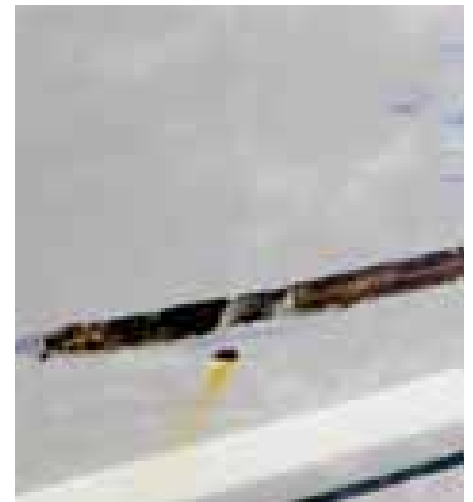
DETAIL OF DAMAGE TO HULL SUSTAINED BY ONE VESSEL.
